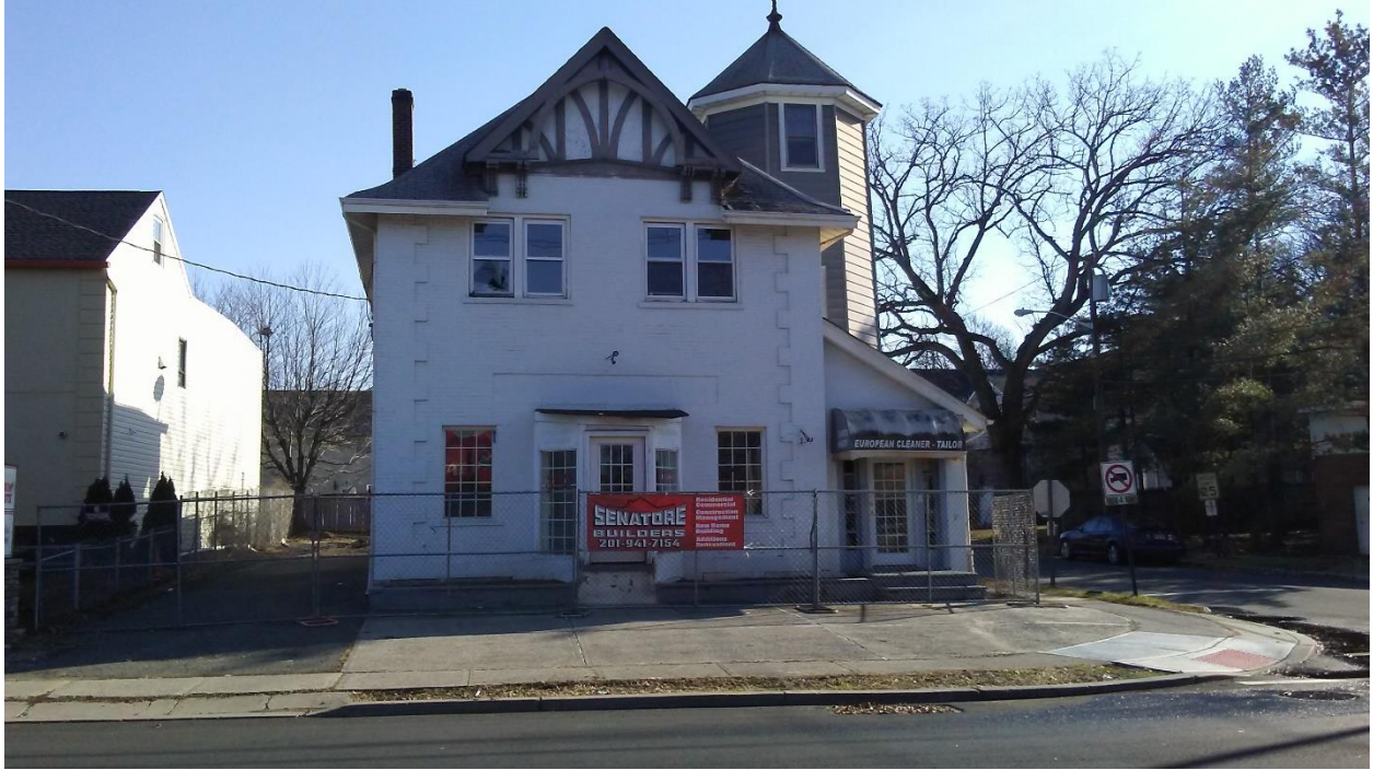
'Nordhoff Firehouse (461 Grand Ave.) shortly before demolition in 2019
